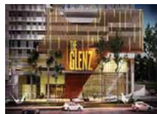
The Glenz Glenmarie Appointed Sales Agent Sg. Besi Construction Sdn Bhd
